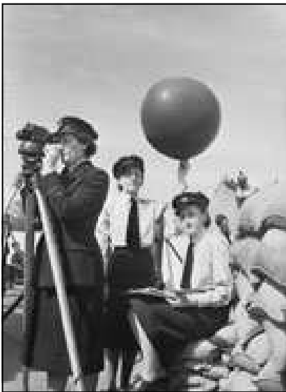
Figure 4 Wartime picture of a balloon tracking theodolite in action.
